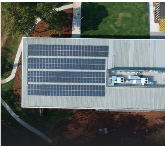
Bracken Ridge Library 100kW Solar PV
