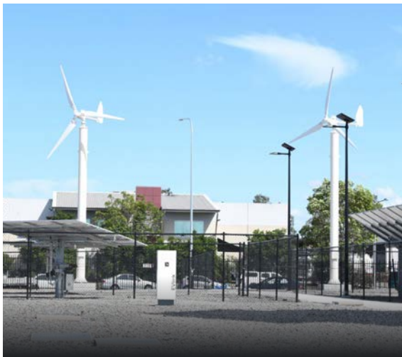
Electrogroup Apprenticeships & Training 100kW Solar, 50kWh Battery Storage, Wind Turbines, Single & Dual Axis Tracking, Solar Carport
