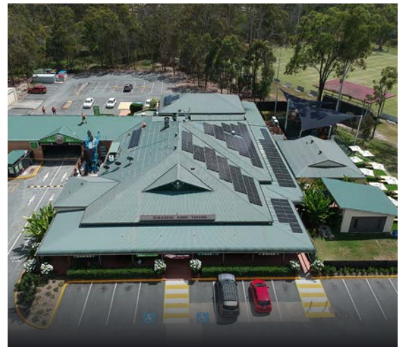
Shearers Arms Tavern 100kW Solar PV
